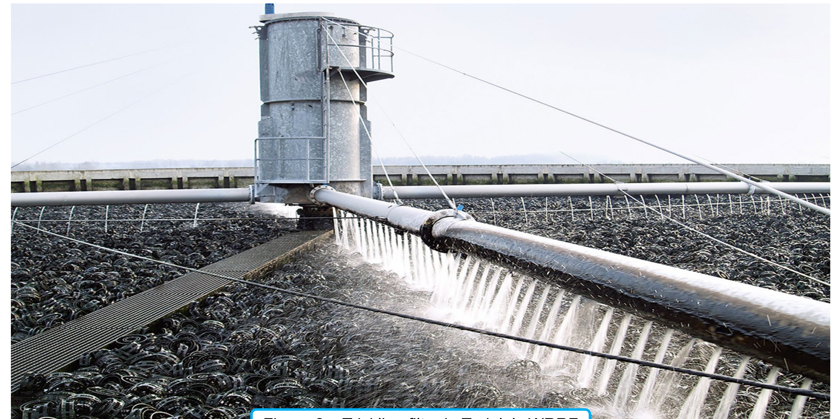
Figure 2 – Trickling filter in Tudela's WRRF
