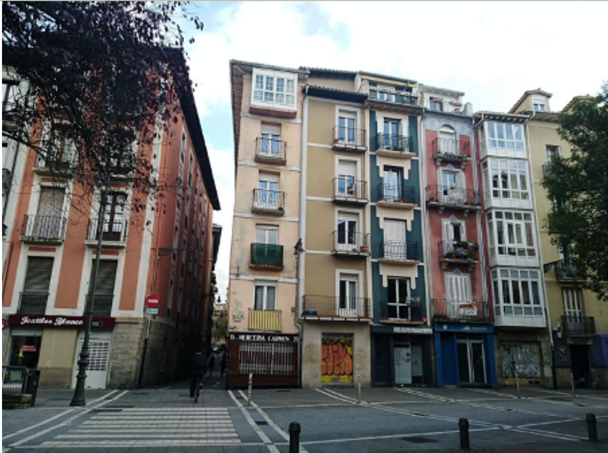
Calle Nueva, by the Plaza de San Francisco. Houses with the typically medieval structure: narrow facades and long deep plans.
